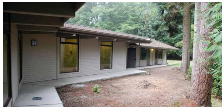
Exterior includes sidewalk to classrooms. Photos courtesy of Wayside UCC.
